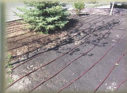
Solar powered, underground drip irrigation.
